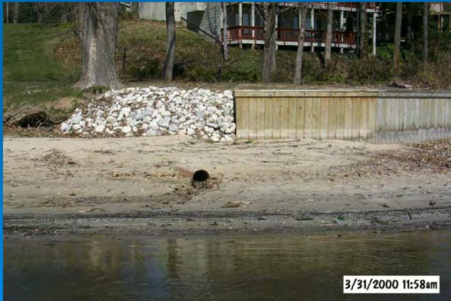
Photo credit: Progressive AE
