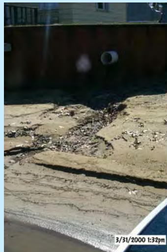
Photo credit: Progressive AE
