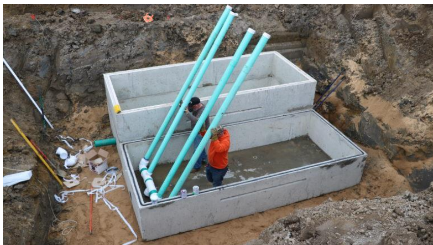
Figure 2. Inlet pipes being laid in the bottom of an iron slag filter. Drainage water enters at the bottom, moves up through the iron slag material (not yet installed) and leaves in a pipe near the top (not pictured) that leads to a nearby surface drain (not pictured). Photo credit: Macatawa Area Coordinating Council.
