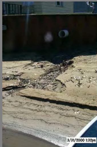
Photo credit: Progressive AE
