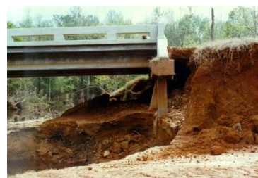
Figure 13. Scour from resulting from bridge placement.
