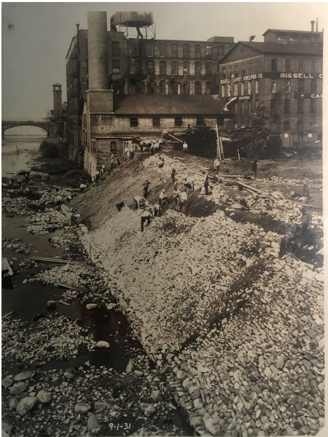
Figure 4 Scrips Program workers grading the Grand River Bank
