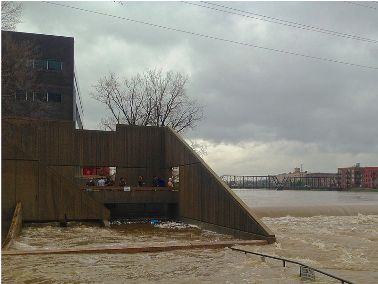
Fish Ladder during 2013 Flood - WikiCommons 4.0 License
