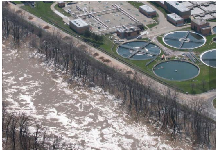
Grand Rapids Water Resource Recovery Facility
