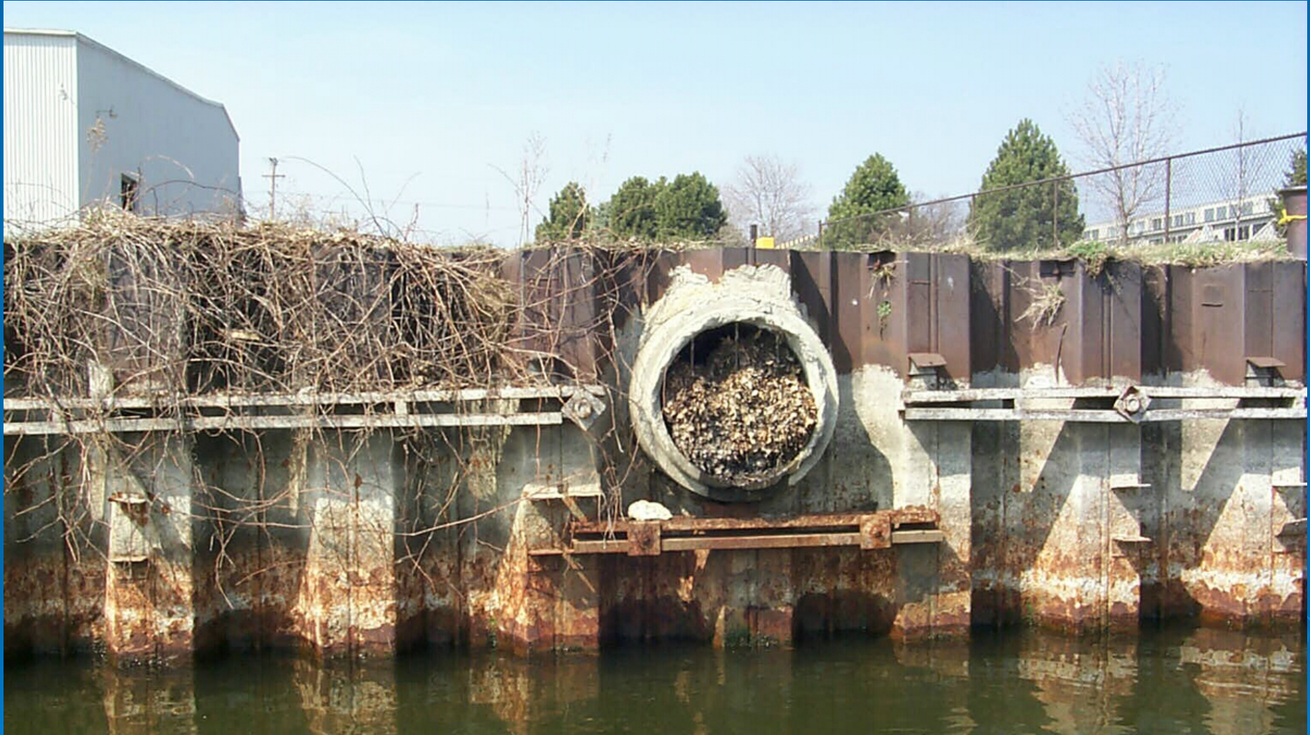
Photo credit: Progressive AE
